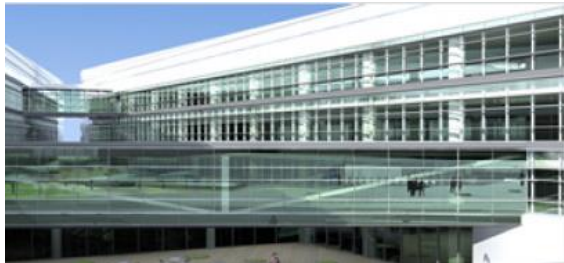
Sancaktepe Engineering Center (2015)
